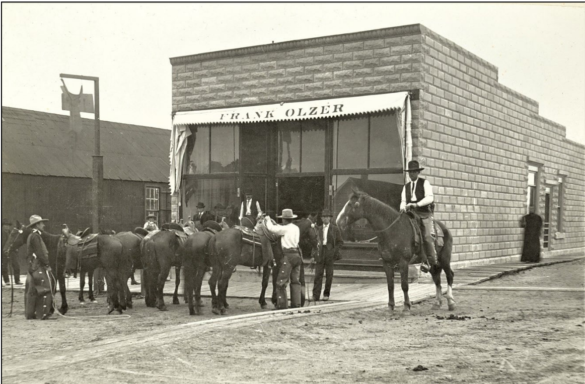
Figure 6. 223 South Gillette Avenue (pre-1918), built by Frank Olzer in 1907 using ornamental concrete blocks. (Campbell County Rockpile Museum)
