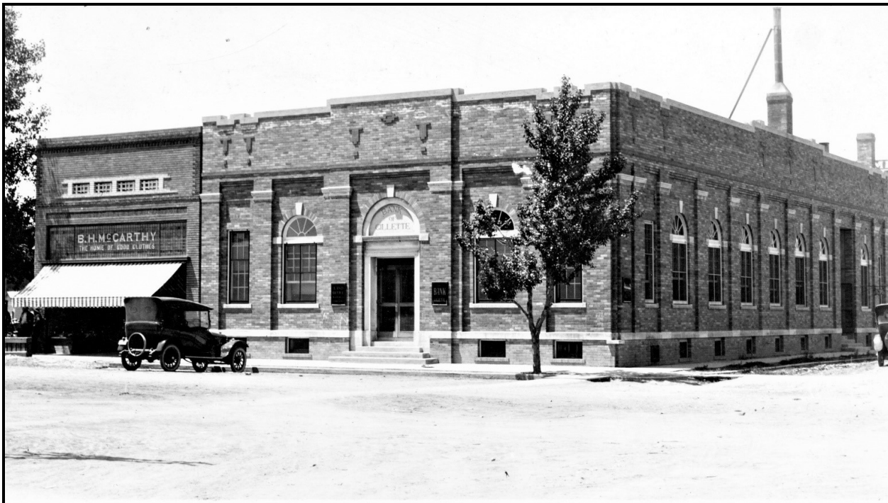
Figure 7. This building was constructed in 1920 to house the Bank of Gillette. It currently functions as a store; the façade has been somewhat altered, but the long north side (at right) remains almost original. This photo dates from between 1920 and 1927. (Campbell County Rockpile Museum)
